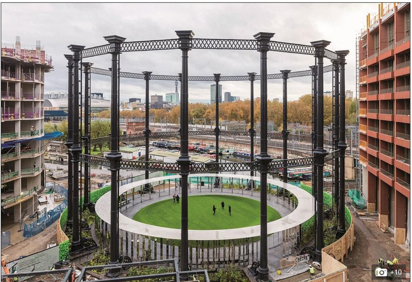
Gasholder Park is a new green space in the heart of King's Cross – a circular lawn that sits inside the carefully restored frame of a Grade II Victorian gasholder, Gasholder No8
